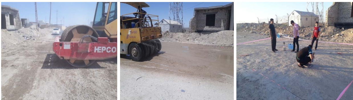
Photo 5. Shows the sprinkle with water, compaction and test the samples
