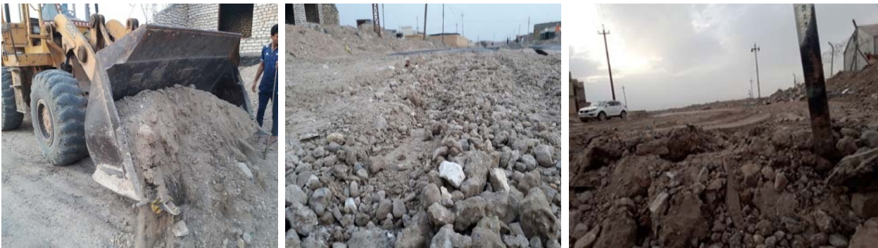
Photo 4. Shows laying the demolition waste subbase for testing
