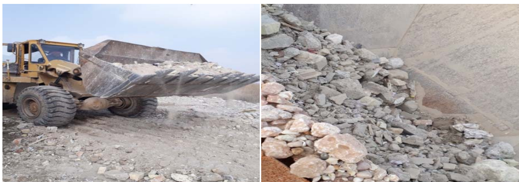
Photo 2. Debris materials Sampling process inside the hopper
