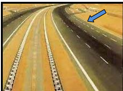
Fig. ( 11 ) One of the High- way parts threatened by sand dunes
