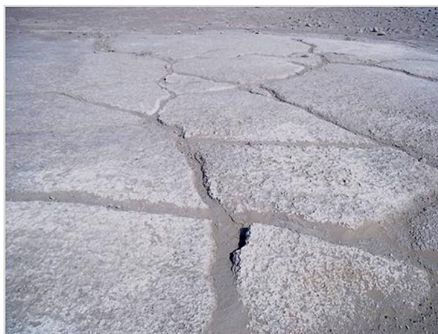
Plate 2- Limestone of Al-Fatha Formation northwest margin of Al-Thirthar lake. Systematic conjugate joints good indication for tectonic activity.
