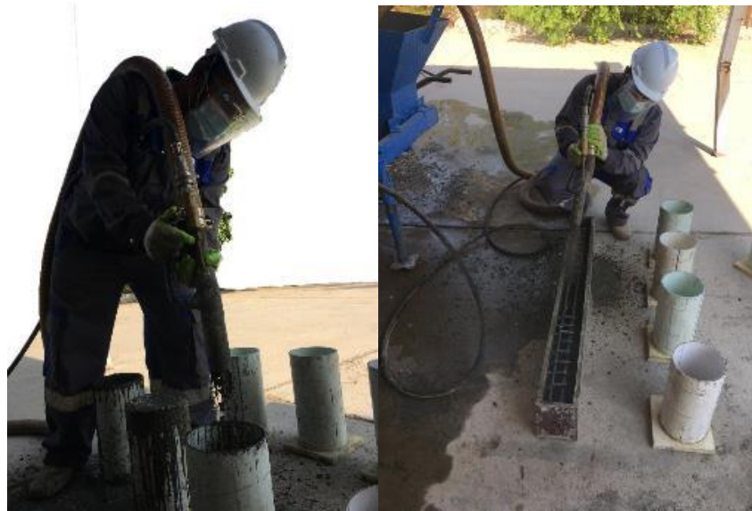
Figure 3-9 Shotcrete casting for hardened properties
