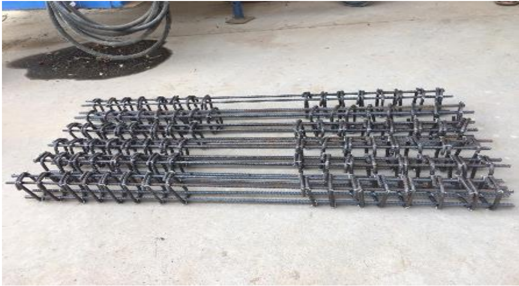
Figure 3-6 Steel reinforcement bars
