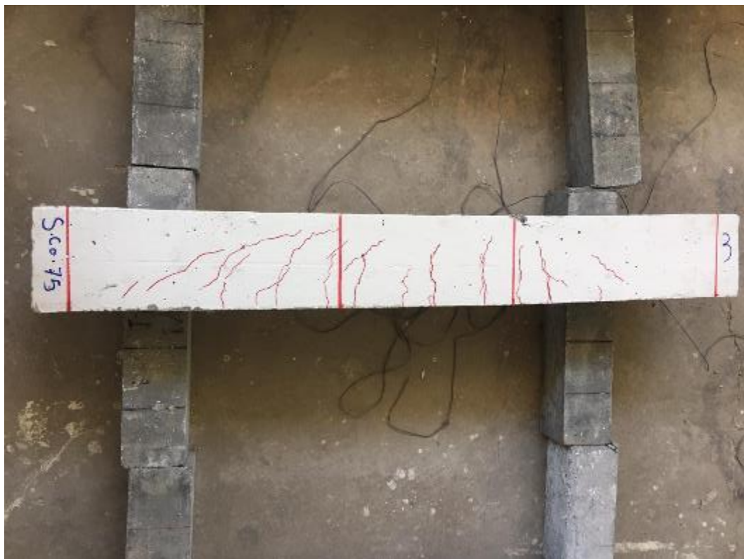
Figure 4-23 Crack patterns of beam SC0.75
