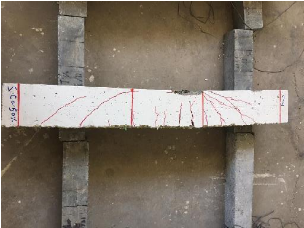
Figure 4-22 Crack patterns of beam SC0.50
