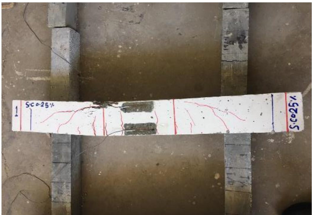
Figure 4-21 Crack patterns of beam SC0.25
