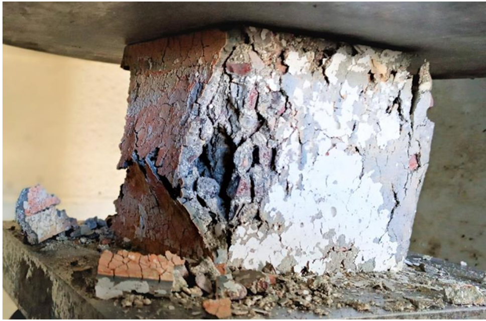
Figure (4-35): The specimen failure at age 90-day under temperature 600°C at 3 hours heating duration.
