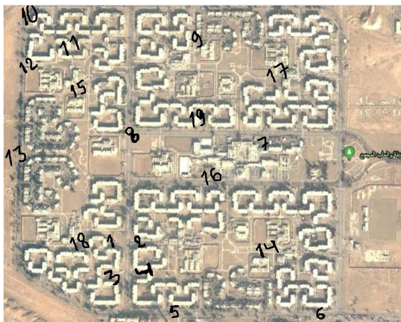
Figure 1. Top view of the Al-door residential complex
