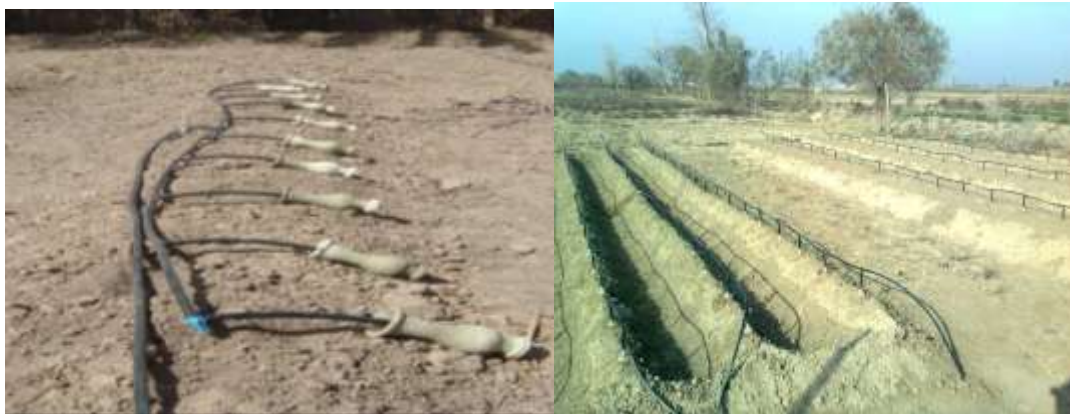
Figure 2. Exudation utensils before burial Figure 3: The exudation irrigation in the case of exudation irrigation system after burying the exudation utensils
