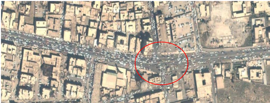
Figure 1.1 Cinema intersection before installing the traffic light
