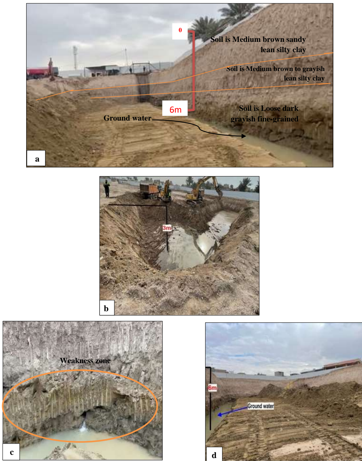
Fig. 3.34: Soil sections of site three.
